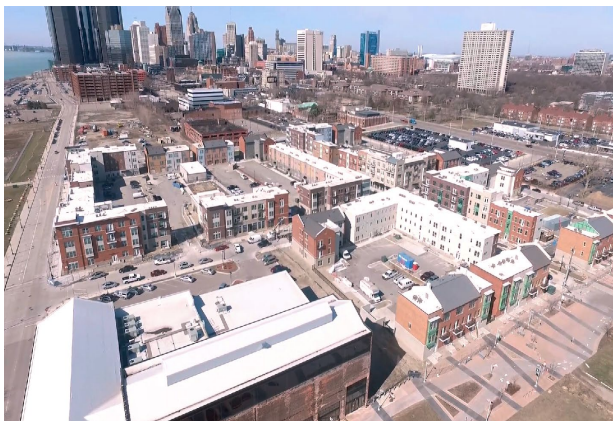
Orleans Landing Redevelopment – City of Detroit
